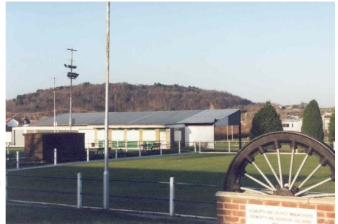
Fig. 3. Dodworth Miners' Welfare - a recreation facility built for miners which is still in use today ( www.hrionline.ac.uk )
