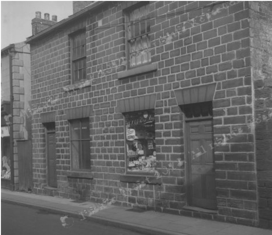
18 and 20 Market Street, Barnsley Demolished for redevelopment in 1962 (The herbalist shop is on the right) © Tasker Trust
