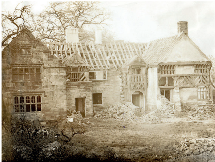
Gawber Hall side A being demolished 1935 courtesy Barnsley MBC
