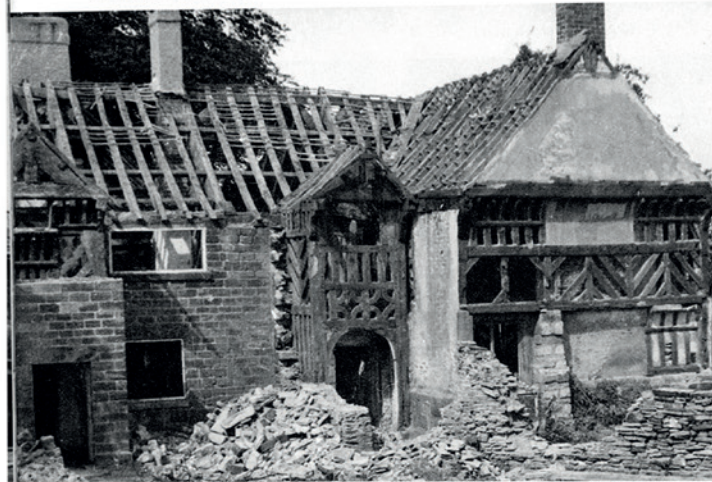
Gawber Hall was situated on a lane connecting Huddersfield Road and Gawber. When the hall was pulled down the interesting timber structure was revealed including a pigeon loft with its numerous nesting holes.
