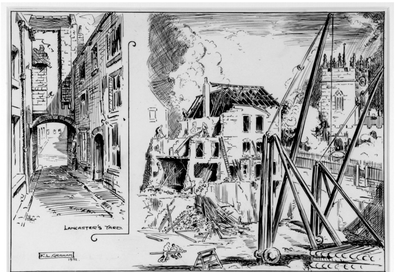
BELOW Demolition/Manor House, Church Street
